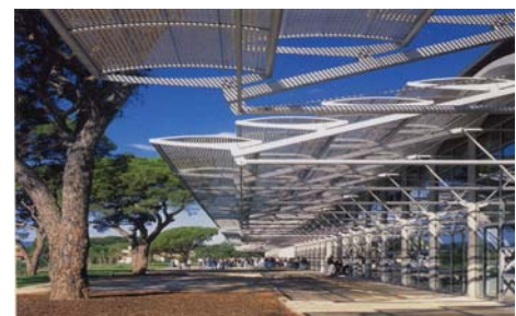
Figure 4: Fixed horizontal shading, Fréjus, France [10]
