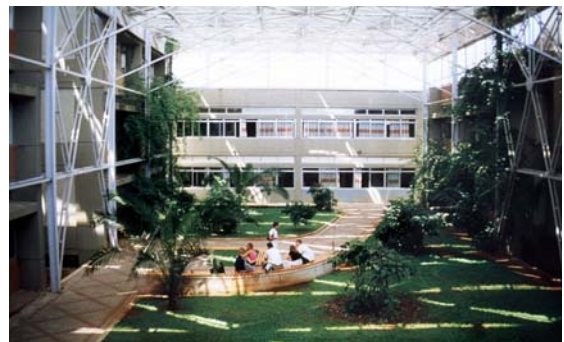
Figure 1: Reduction of overheating by passive strategies Retrofitting, University of Ioannina, Greece [11-13]
