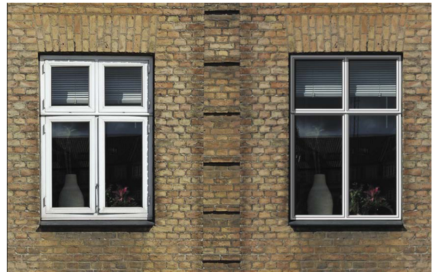
Figure 33. The new GRP window shown to the right alongside a window from the 1980s.
