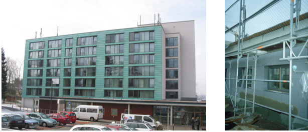
Figure 72: Photos of the retrofitted nursing home in Stuttgart-Sonnenberg (left) and of the application of the graphite embedded EPS-system (grey) on the south and north side of the building (right).
