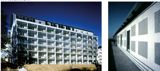
Figure 73: Photos of the multi-family house in Munich (left), and of the application of transparent insulation at the exterior wall of the top floor (right).
