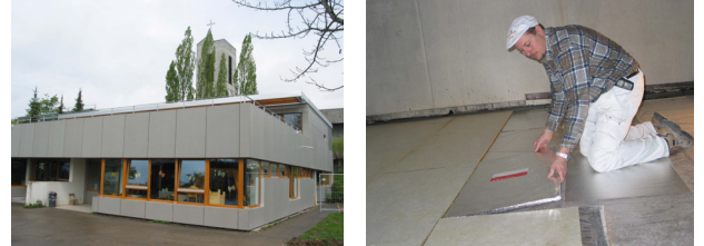
Figure 74: Photo of the retrofitted community centre in Ulm (left), here kindergarden, and of the application of vacuum insulation panels at the floor of the kindergarden (right).
